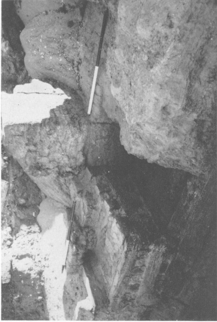
1. Detail of postern gate in Area 1, seen from NW, showing three phases of construction
